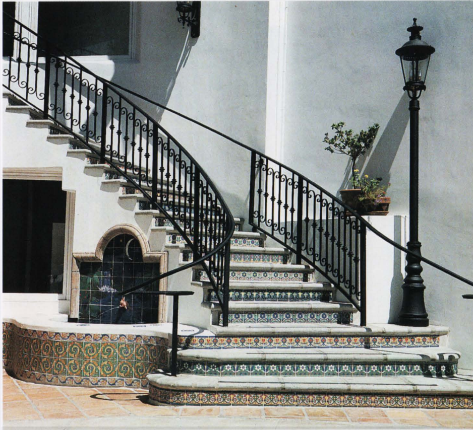
◀ 124 New decorative tiles, inspired by traditional California tilemakers, accent the risers of this beautiful outdoor stair.
